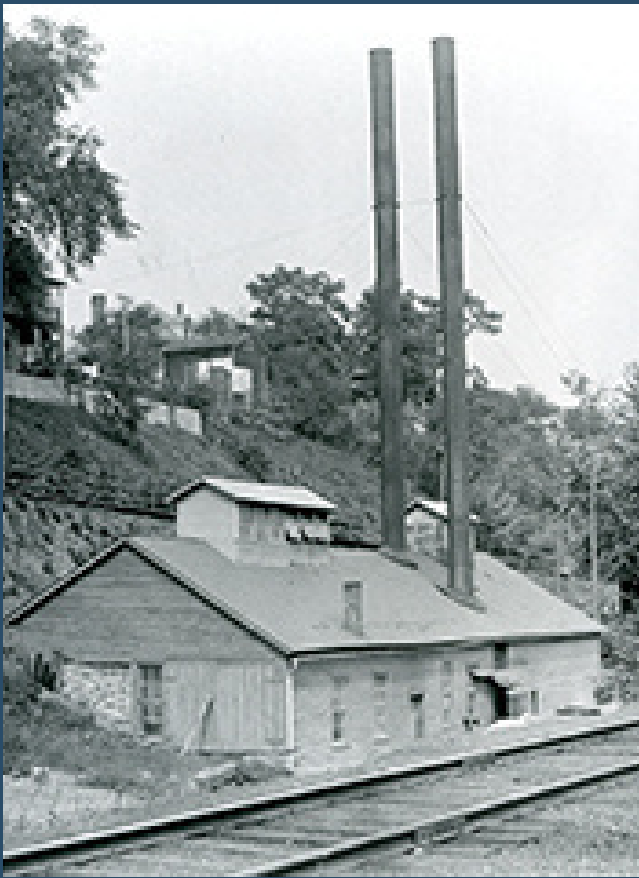
Berwick Water Company Plant, 1920
