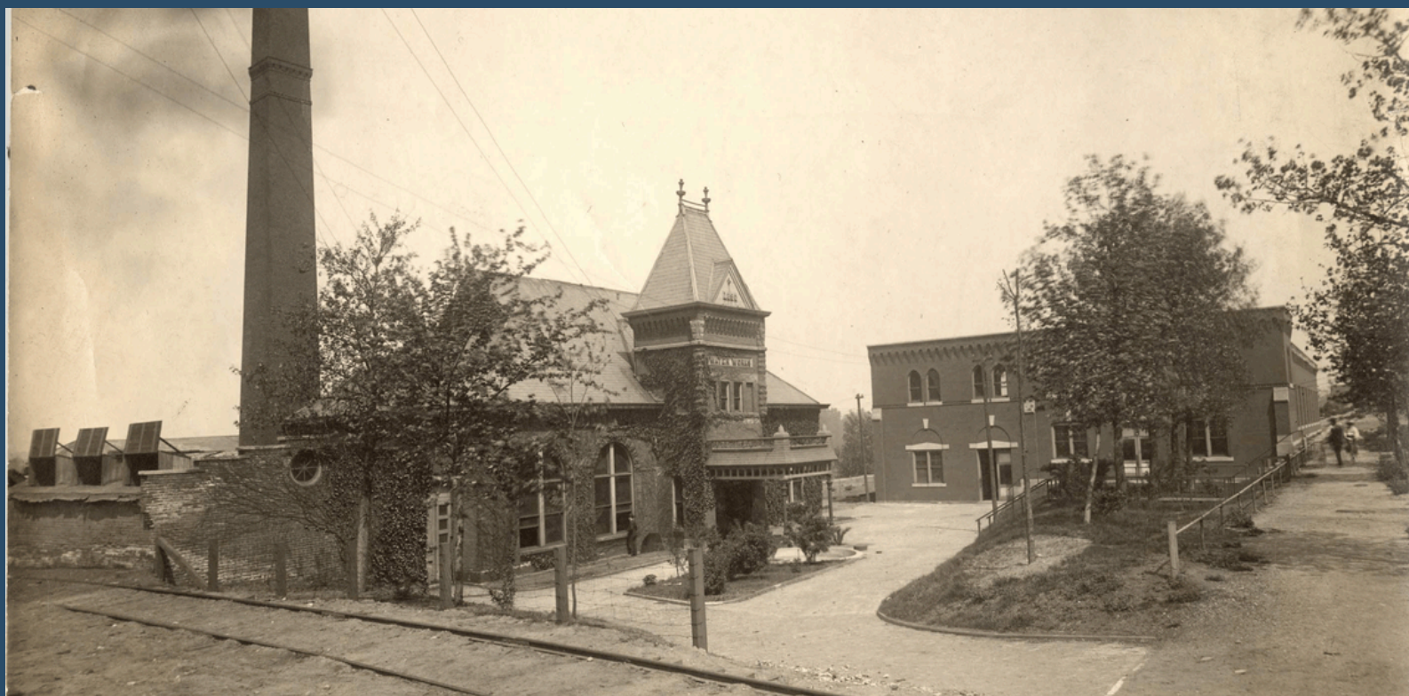
Terre Haute Water Works Main Station, 1912
