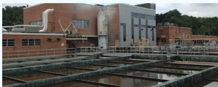
More than $8 million is being invested in the Scranton wastewater treatment plant headworks to improve performance and reliability.
